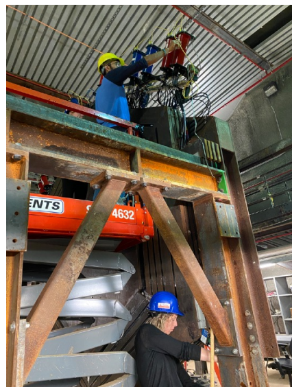
PMT/FEB installation and cabling
