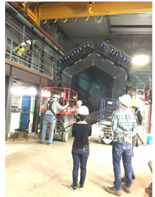
Safety review of PMT repair scheme
