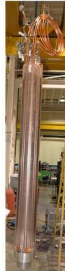
Water lines in place
