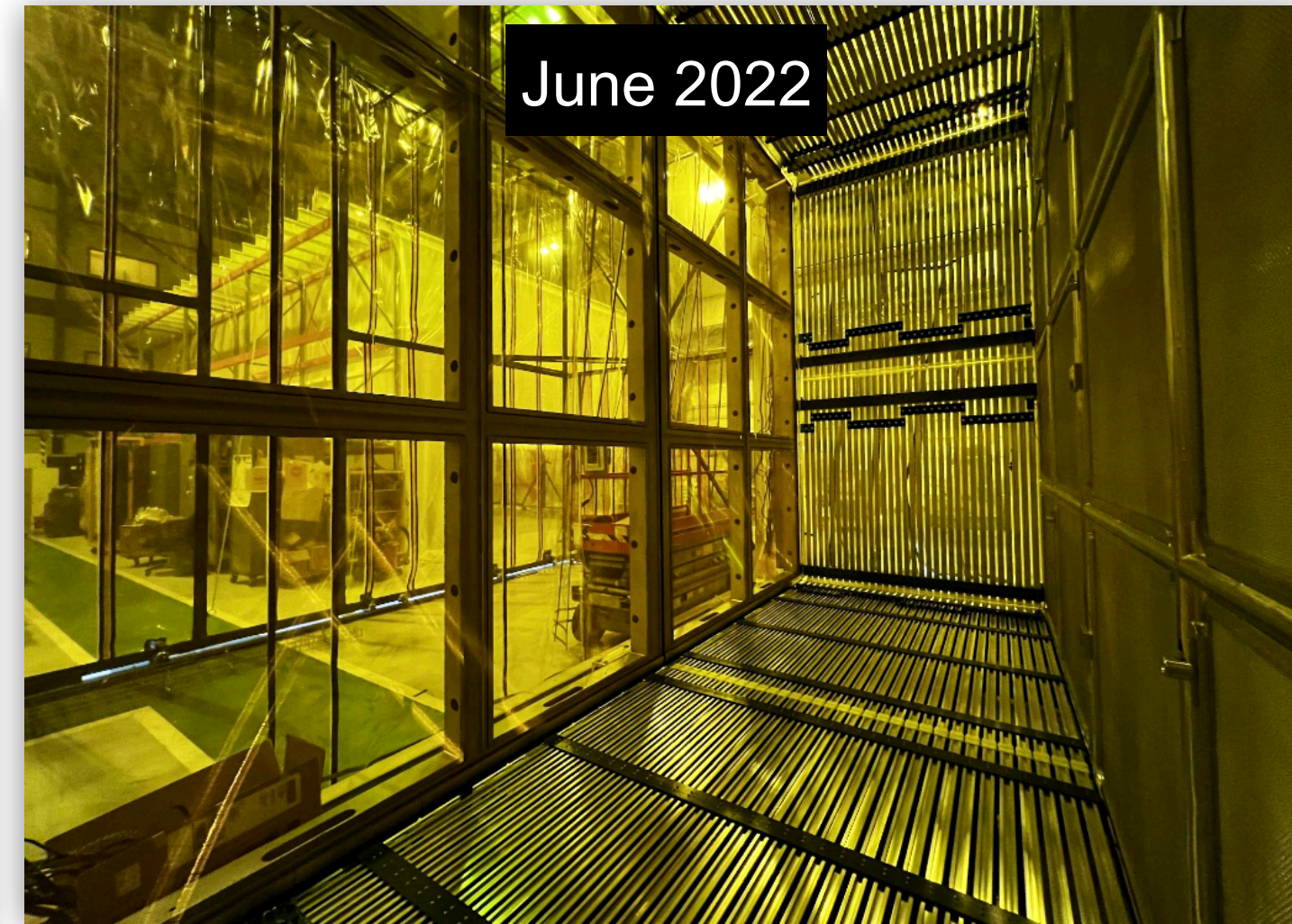
Installation of field cage completed
