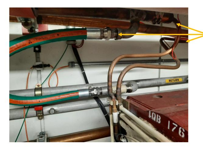
CONNECTIONS FROM QUAD BUS TO MANIFOLDS AND MAGNETS WILL MOVE WITH RELOCATED BUS DOWN TO NEW LOCATIONS
