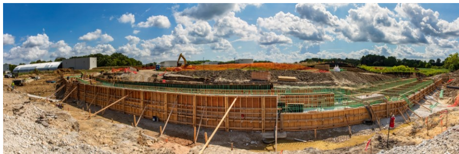
New culvert system (with fish channel) to reroute Indian Creek
