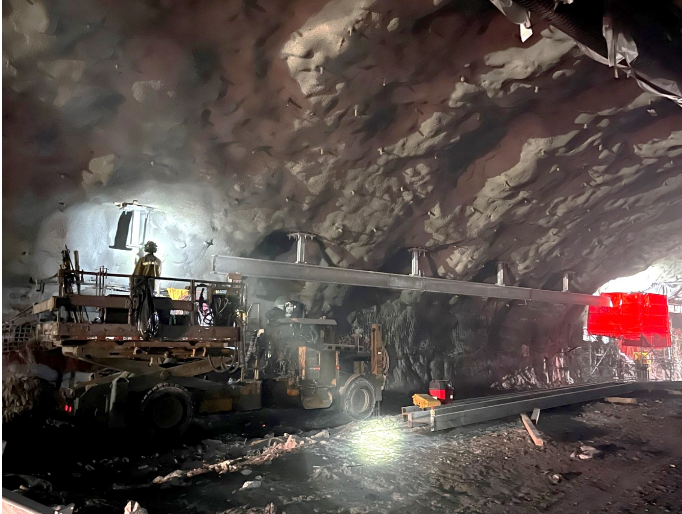
Extending monorails that will support material handling cranes in South Detector Cavern (4850-37)
