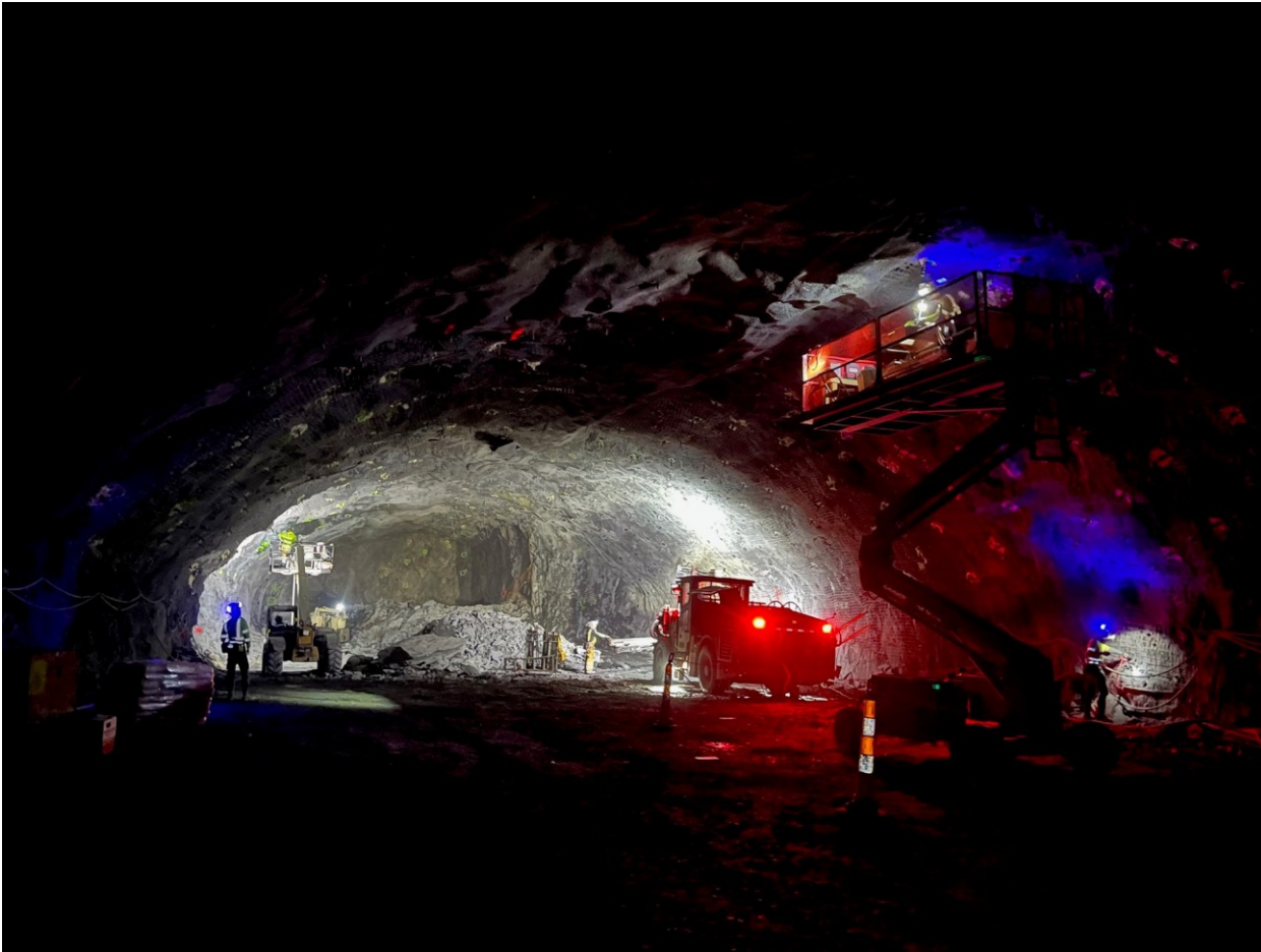
Finishing Cut 2 and testing Rock Bolts in Central Utility Cavern (4850-36)
