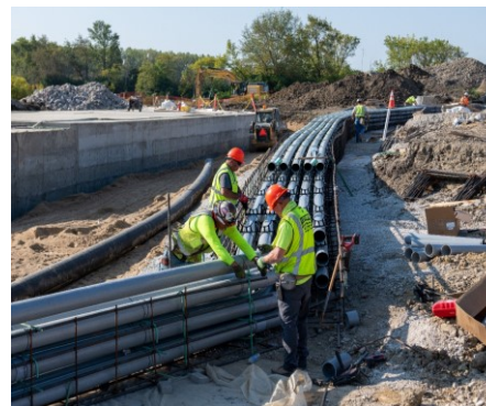
Power distribution system installation
