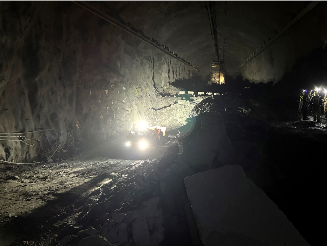
Removing blasted rock for bench D in North Cavern (4850-33)
