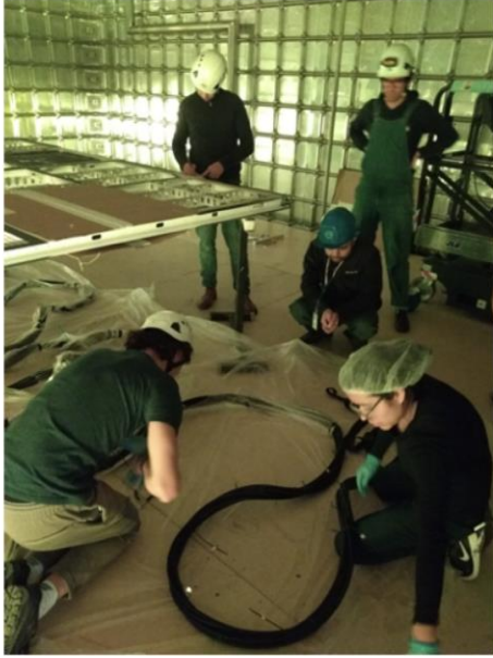
Figure 27. Fiber bundle moved to cathode at <math><2\text{m}</math> working height for routing on cathode.
