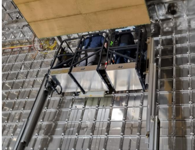
Figure 15. Dual scissor lift installation approach for membrane suspension system work.
