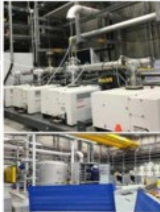
Compressors and Oil Removal System (WCS)
