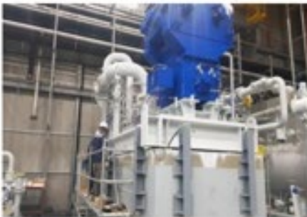
Compressors and Oil Removal System (WCS)
