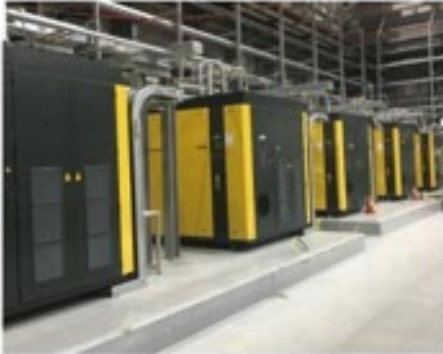
Compressors and Oil Removal System (WCS)
