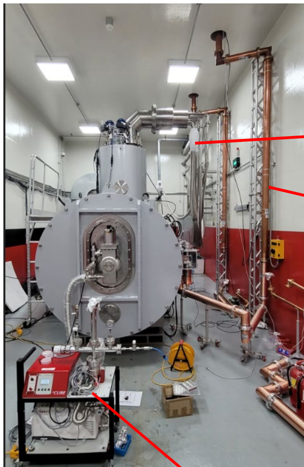
Vacuum pump for cavity
