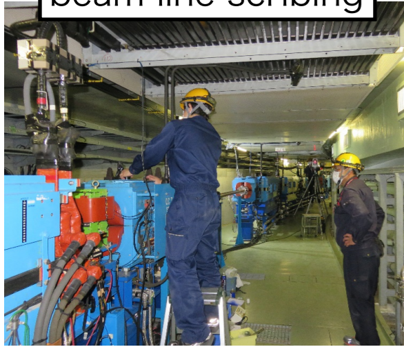
Transfer and installation of dipole magnet
