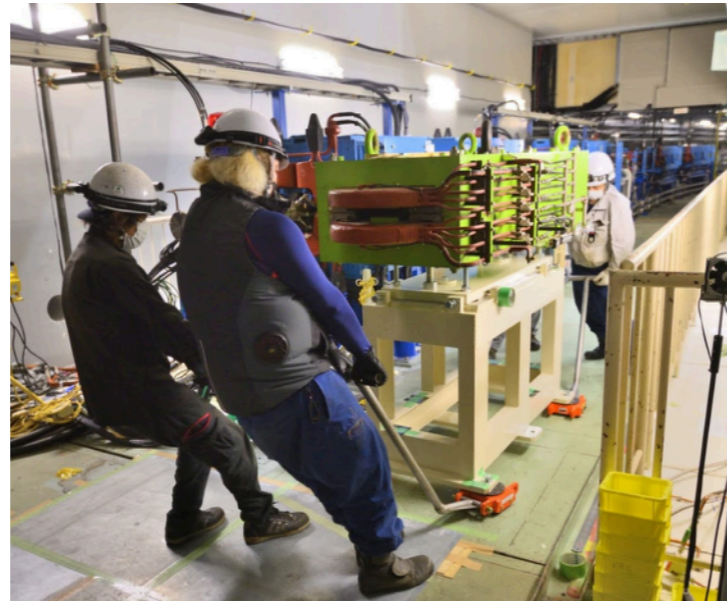
Transfer and installation of dipole magnet
