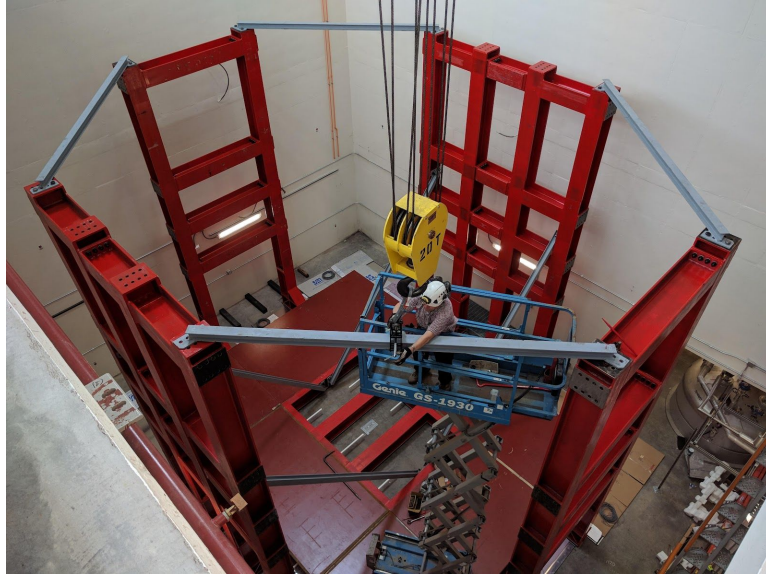
Oct/Nov '19: cryostat steel support structure installation
