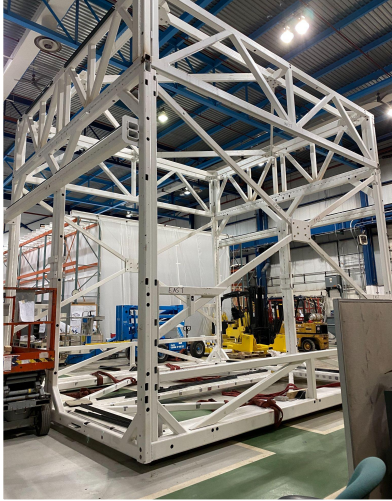
Fall 2019 - Assembly Transport Frame Construction
