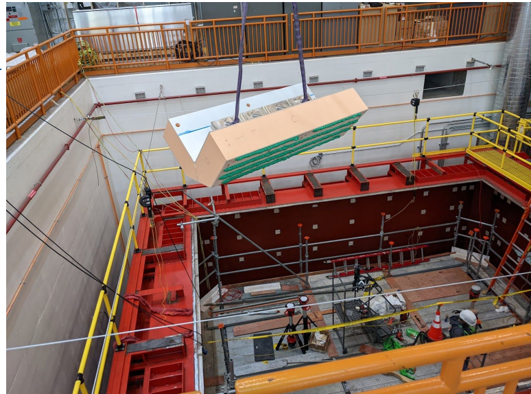
May/Jun '22: cryostat insulation installation
