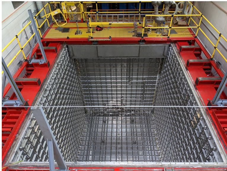
Jul/Aug '22: stainless steel membrane installation
