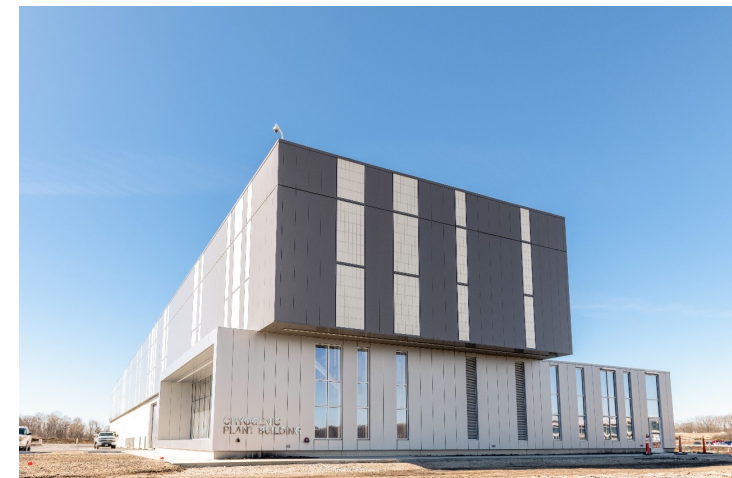
Cryogenics Plant Building is complete
