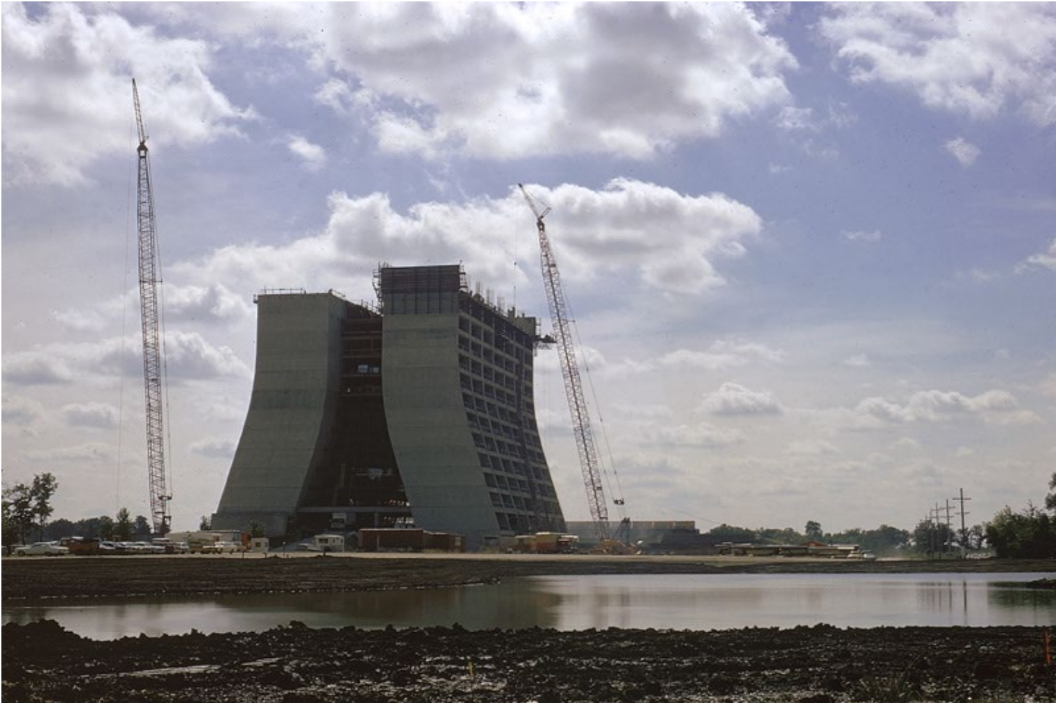
Construction of Wilson Hall began in 1971.
