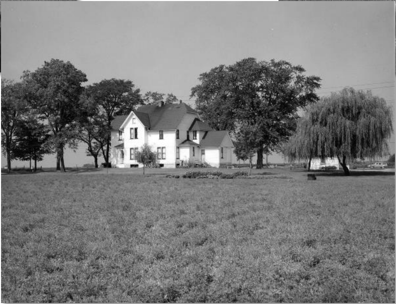
Some of the other houses and barns on the site.
