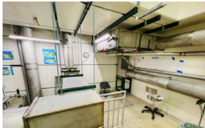
Cryogenic feedboxes and transfer line installations complete
