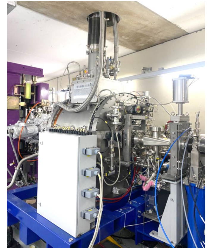
Cryomodule in SSRF tunnel
