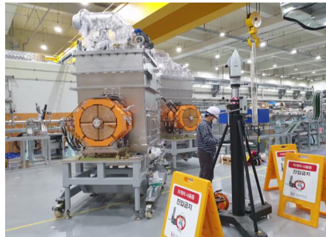
⑤ Alignment between warm sections and cryomodule
