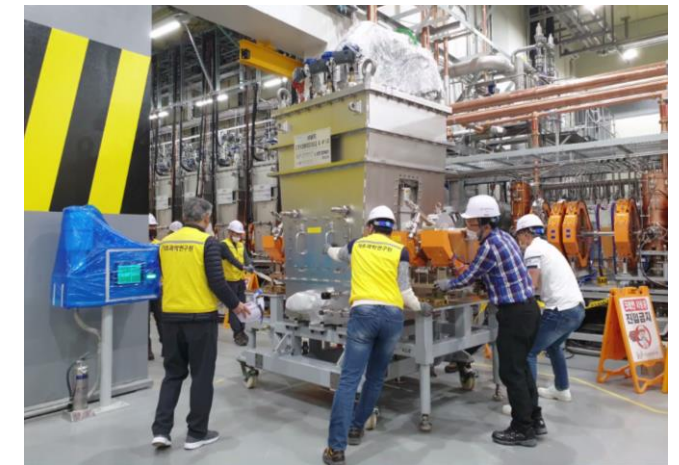
⑥ Moving CM into the tunnel, then install it
