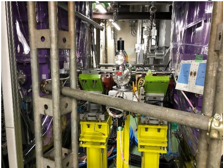
Installation of lower half of Q-mag.
