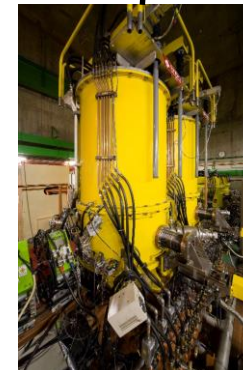
RIKEN Heavy-Ion Linac (RILAC) Facility
