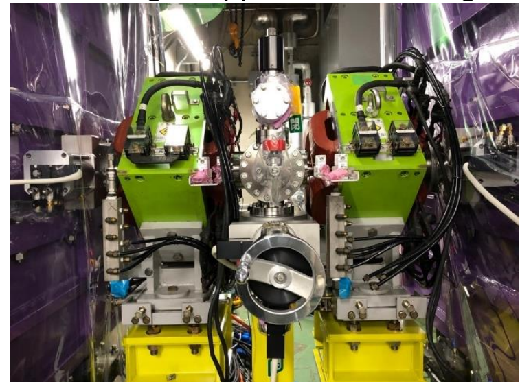
Mounting of upper half of Q-mag.
