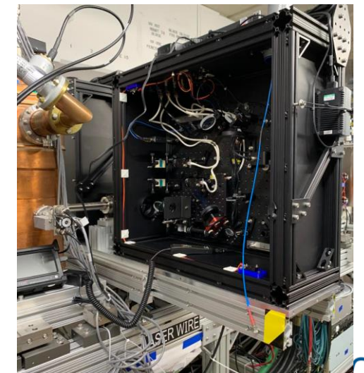
System Commissioning at PIP2IT
