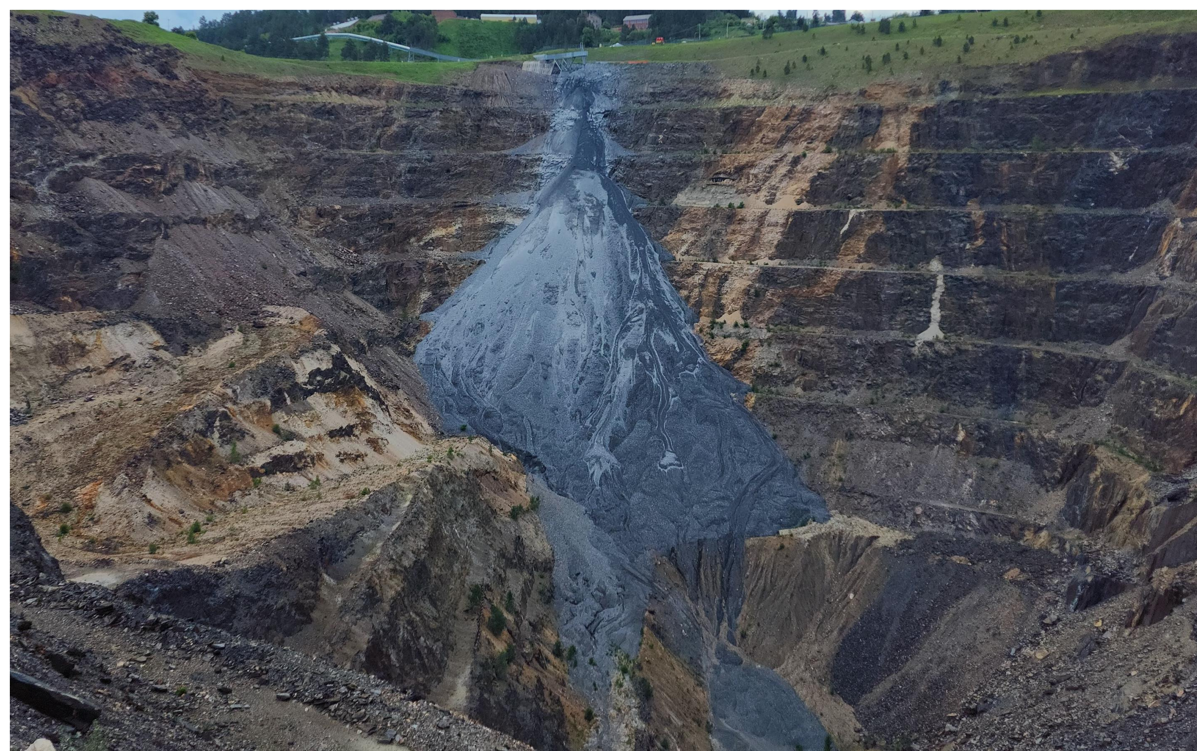
Figure 1 – Image of the Open Cut and discharged rock on July 3rd, 2023.
