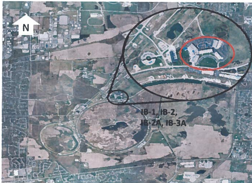
Technical Division Industrial Complex
