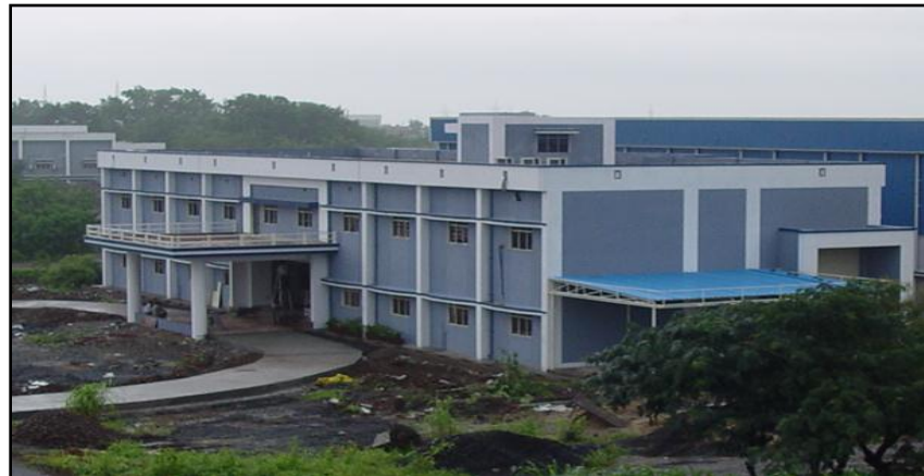
Test and measurement facilities building
