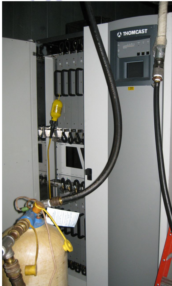
Refurbished 162.5 MHz VHF TV transmitter Water cooled Thomson 10 kW Solid-state
