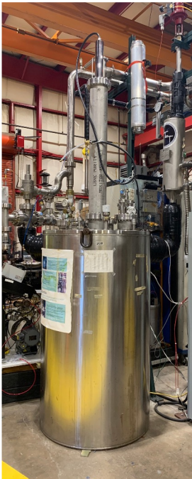
HV FT Test Setup in BLANCHE @NLTF
