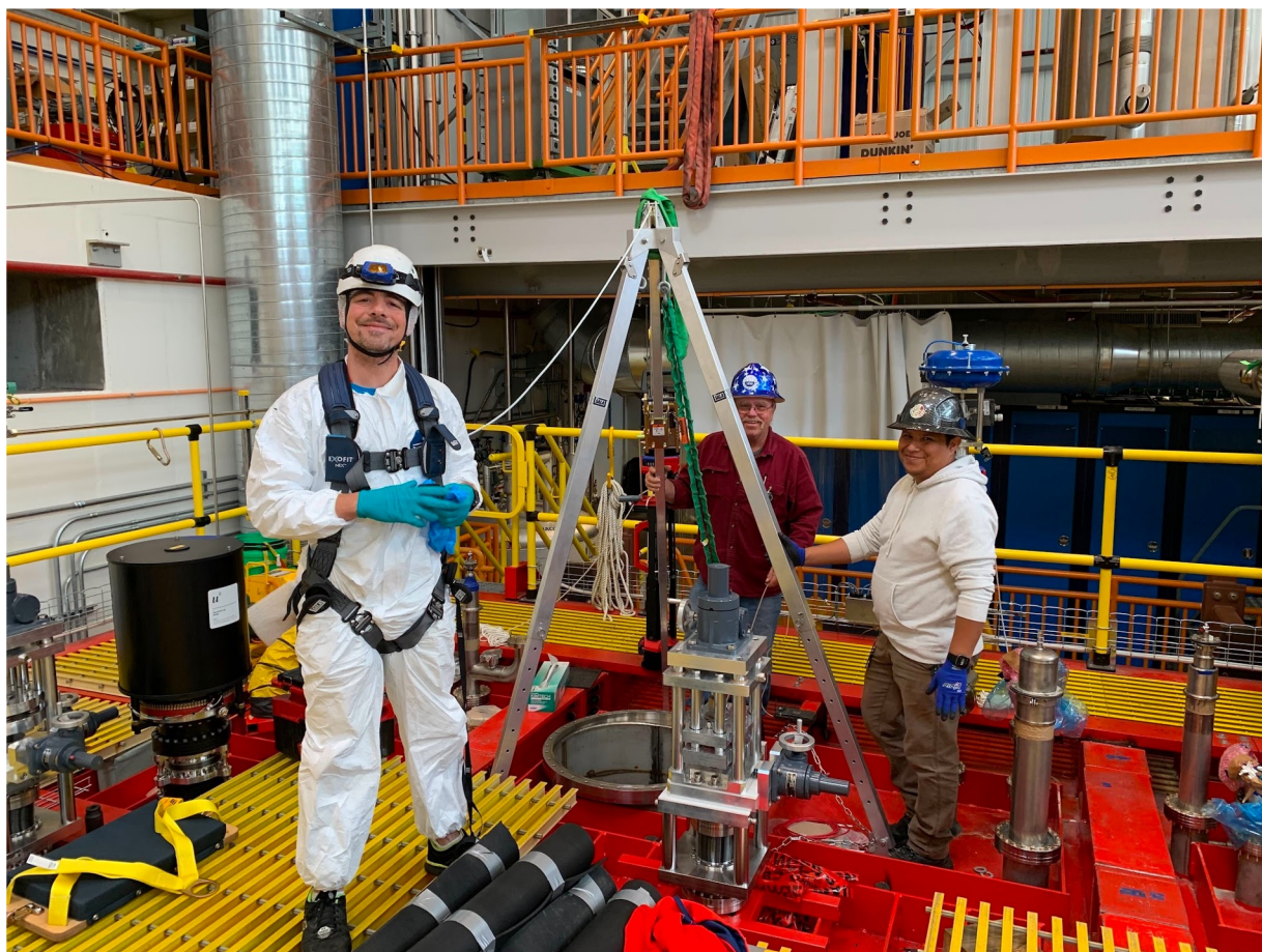
Access to the inside of the cryostat through an access port on the cryogenics top cap using a bosun's chair
