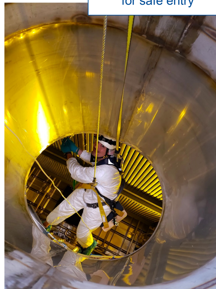
Access to the inside of the cryostat through an access port on the cryogenics top cap using a bosun's chair
