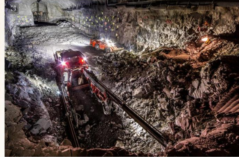
A drill and mucker are seen excavating for the Deep Underground Neutrino Experiment at the 4850 Level at SURF. Photo by Matthew Kapust, Sanford Underground Research Facility Matthew Kapust
