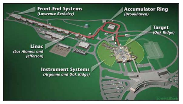
The SNS is putting 2x10<sup>23</sup> ~1GeV protons on a liquid Hg target per year (1.4MW).
