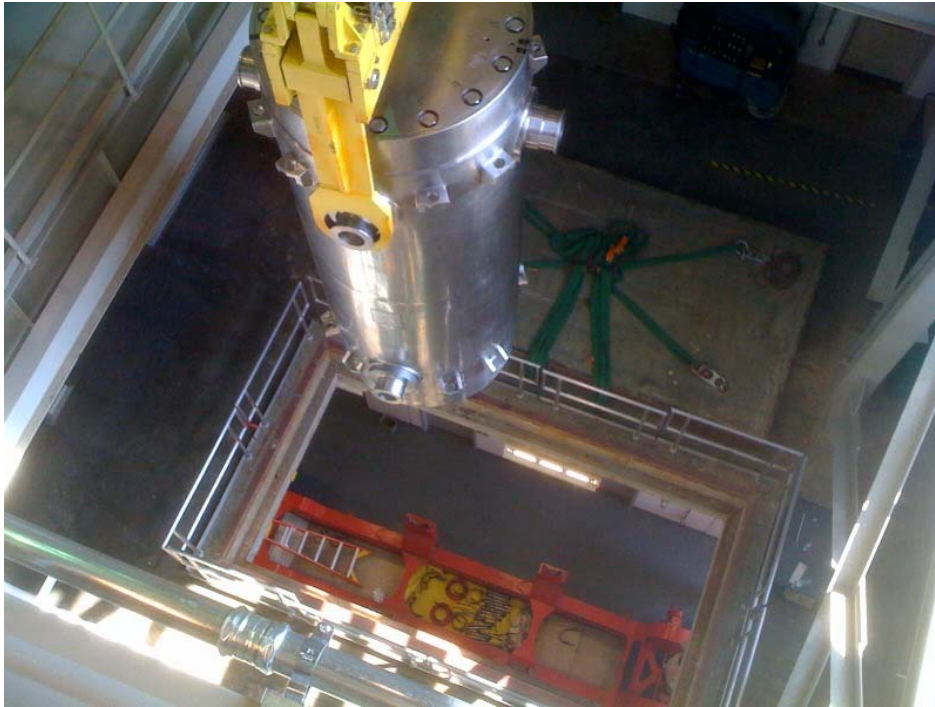
Cask Lifting from Truck
