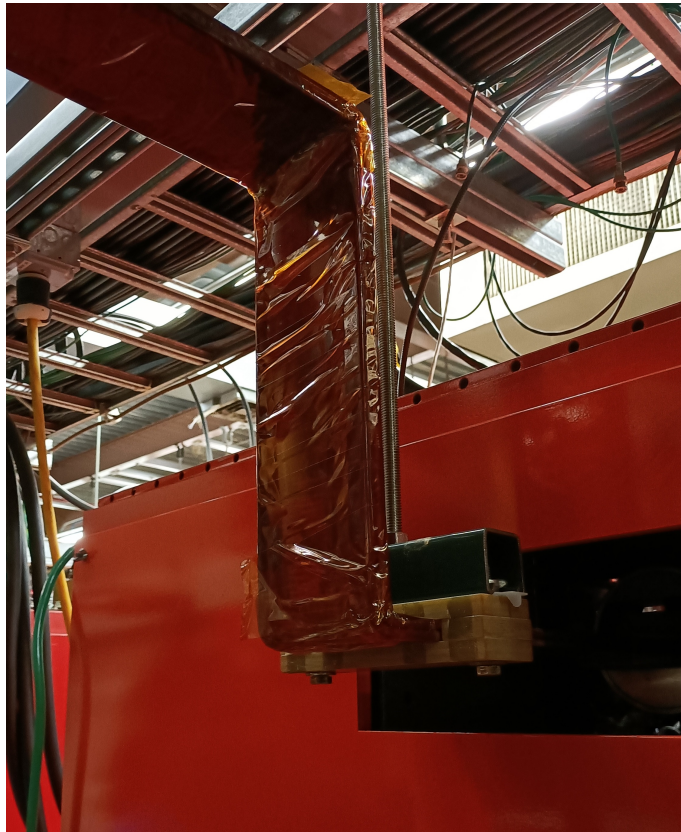
Figure 8: Bus bars behind the bias supply
