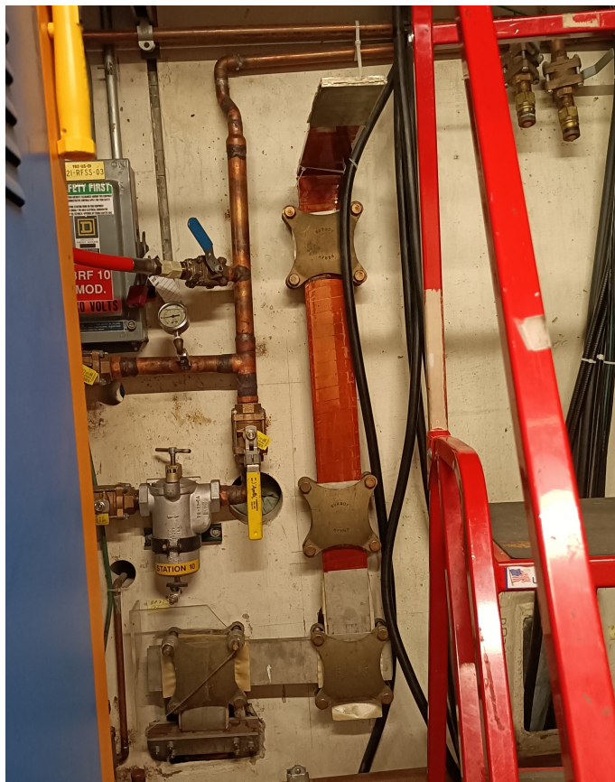
Figure 9: Bus bars as seen from the gallery (Booster station 10)
