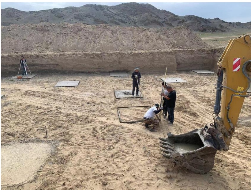
Underground Pier 1.6m*1.6m
