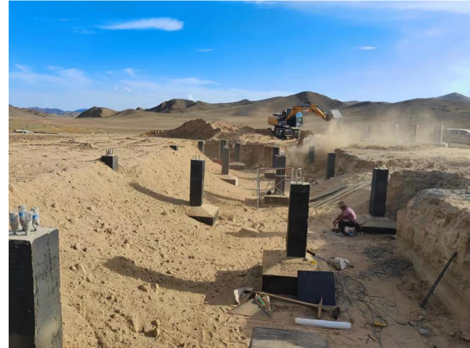
Backfill the soil
