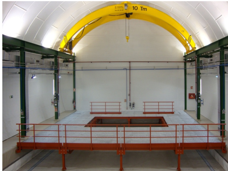
Current view of main laboratory hall with completed work platform.
