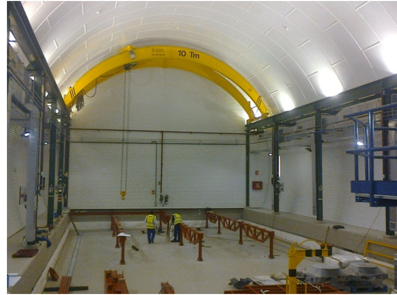
View of main laboratory hall during the platform installation.
