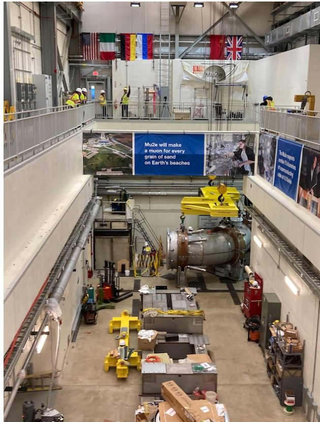
TSu lowered to pit
