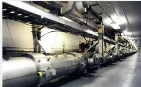
Cryomodules in the accelerator tunnel
