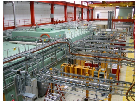
FAST Facility under construction in repurposed NML building
