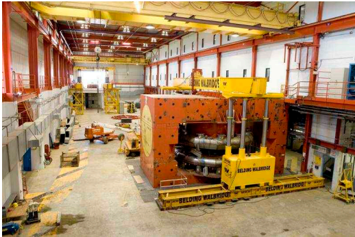
NML During Removal of Chicago Cyclotron Magnet(CCM) (2006)
