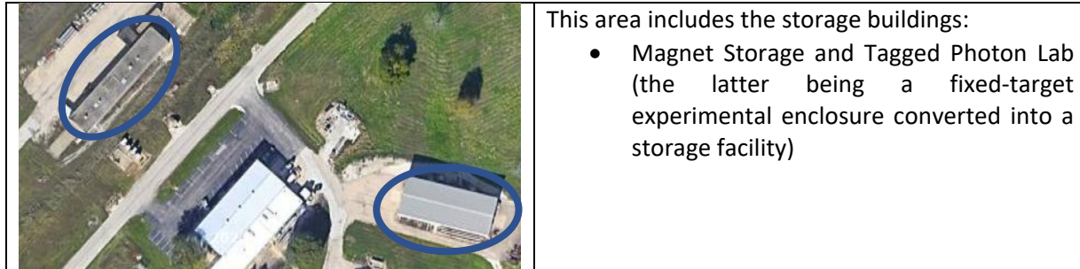
Figure 3. Aerial close-up views of the APS-TD facilities.
