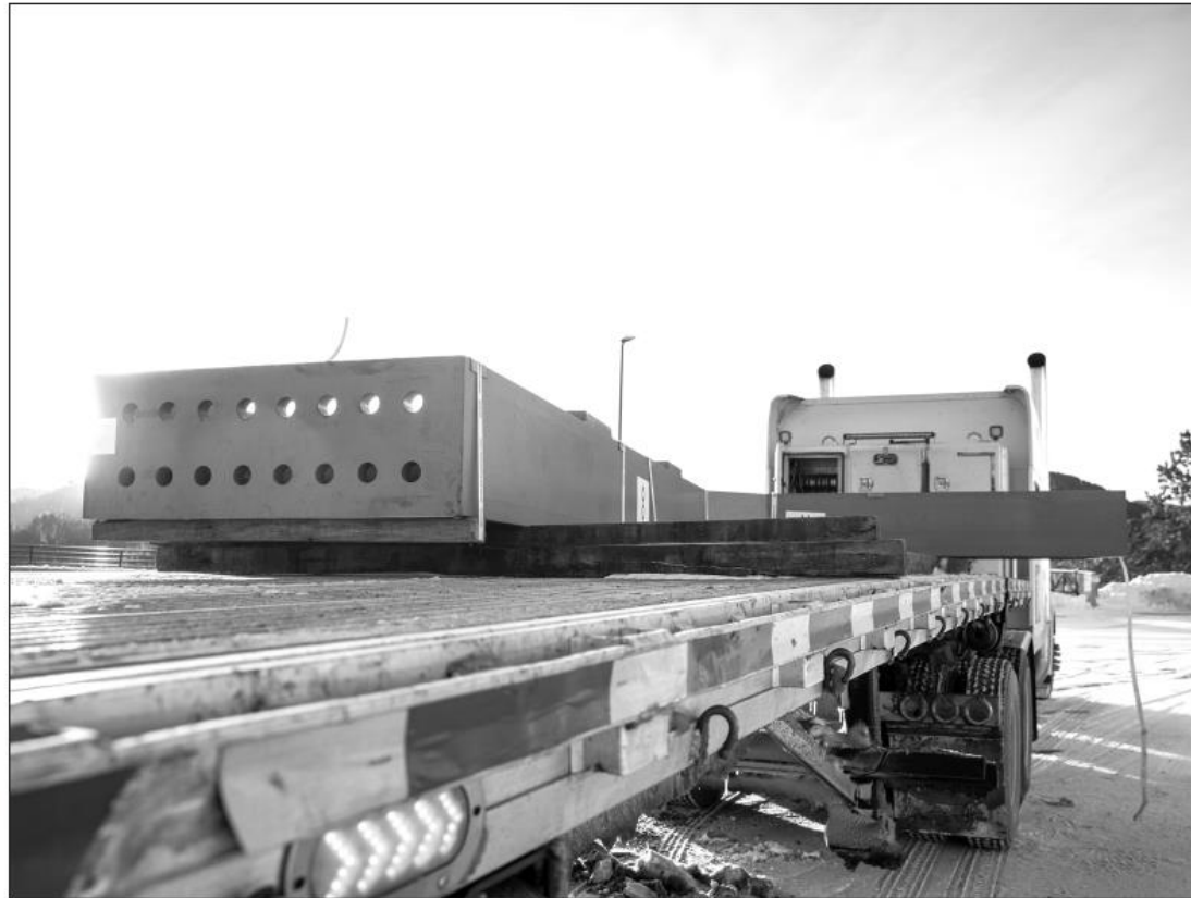
This L-beam is nearly 6 tons and will form a corner of a massive cryostat after it is lowered 4,850 feet down the Ross Shaft. Photo by Stephen Kenny
