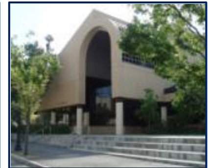
Stanford Nano-Fabrication Facility
