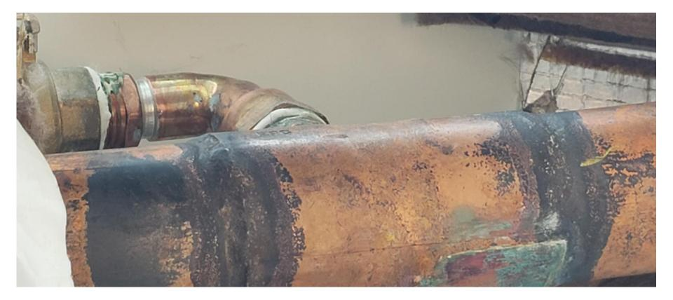
Behind the 1.5 Inch Brazed Copper Pipe is an elbow with a threaded connection. It may be that the treaded connection is where the leak occurred as a plastic cup is placed below the threaded connection.
