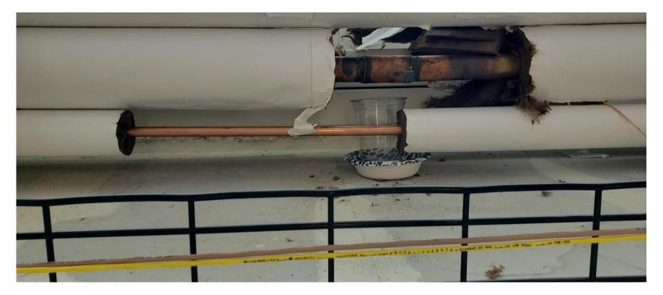
1.5 Inch Brazed Copper Pipe for heating located above office 1770 (IERC West Side, Upper Level). Appears to be very poor quality braze joint with perhaps a patch (see next slide). This should not have been accepted by the construction management people.
