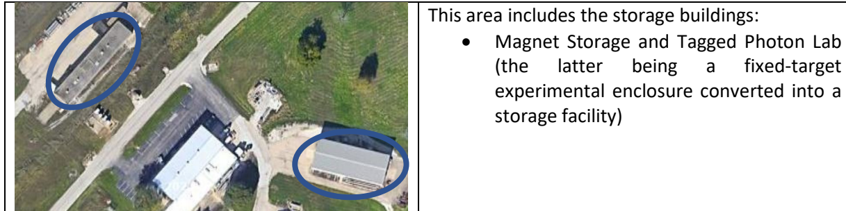
Figure 3. Aerial close-up views of the APS-TD facilities.
