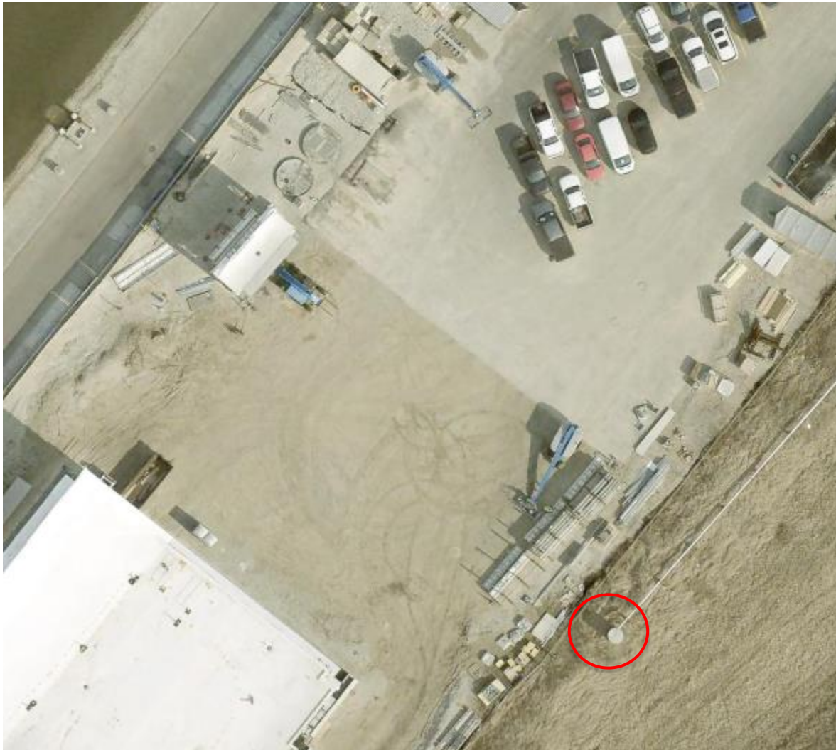
Figure 1: Location of the Enclosure B cryo penetration located on the berm adjacent to the Helen Edwards building.
