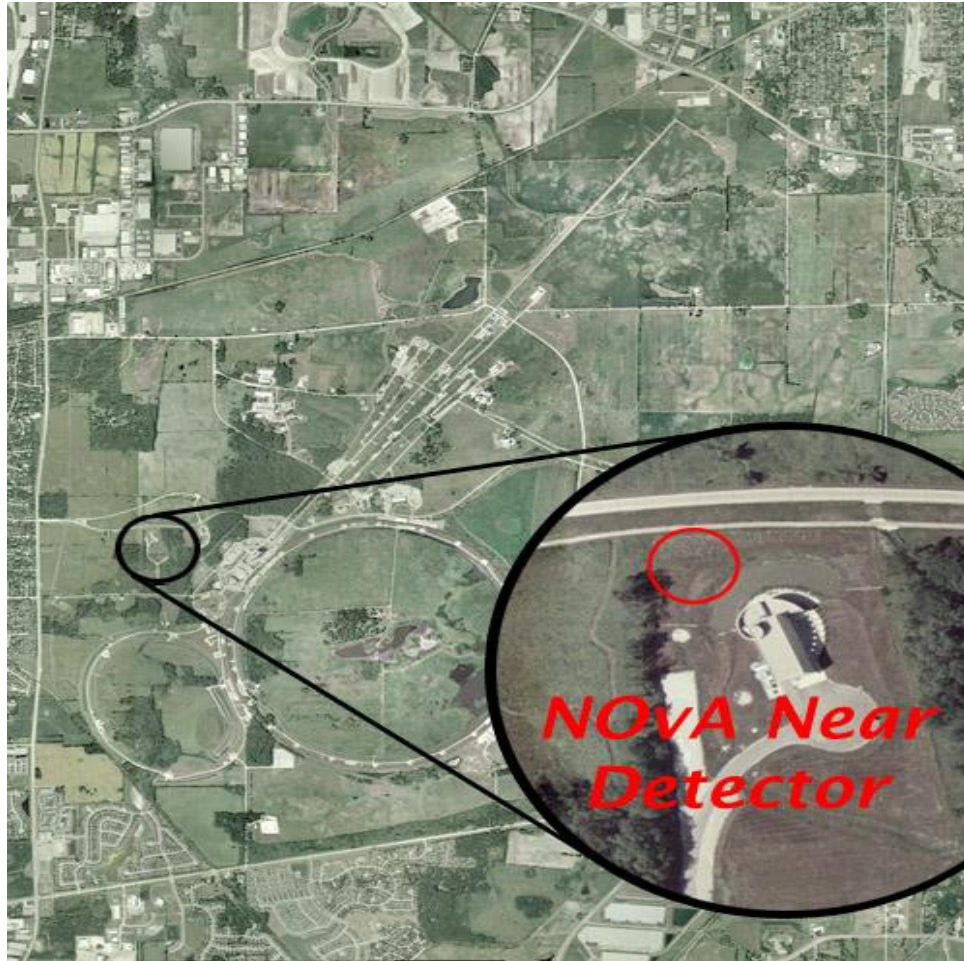
Figure 3. Aerial view of the Fermilab site, indicating the location of the NOvA Near Detector.
