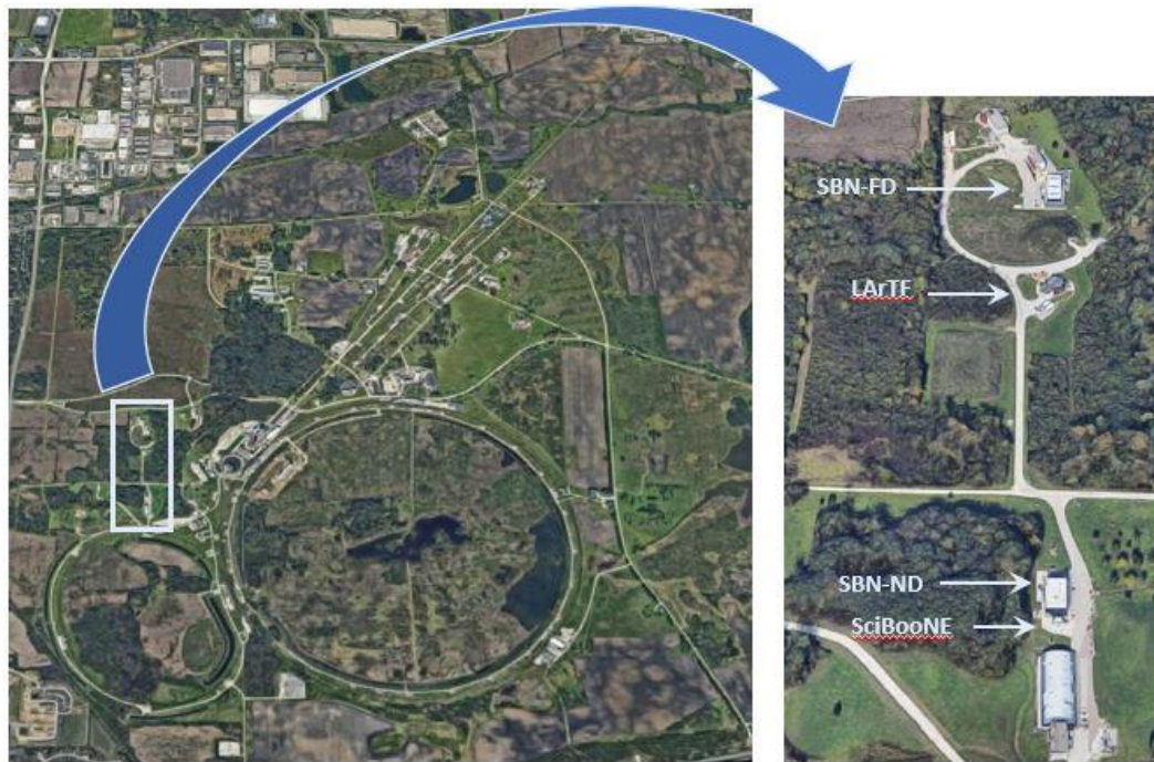
Figure 2. Aerial view of the Fermilab site, indicating the location of the SBN Experiment Areas.
