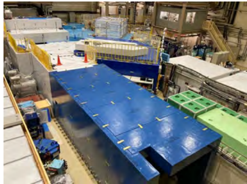
Beamline under Construction
