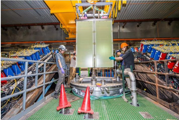
4 modules of the 2x2 hanging above the cryostat during installation
