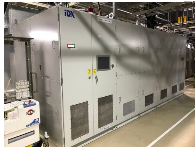
New Horn PS/ trans/strip-lines for 320kA, 1Hz
