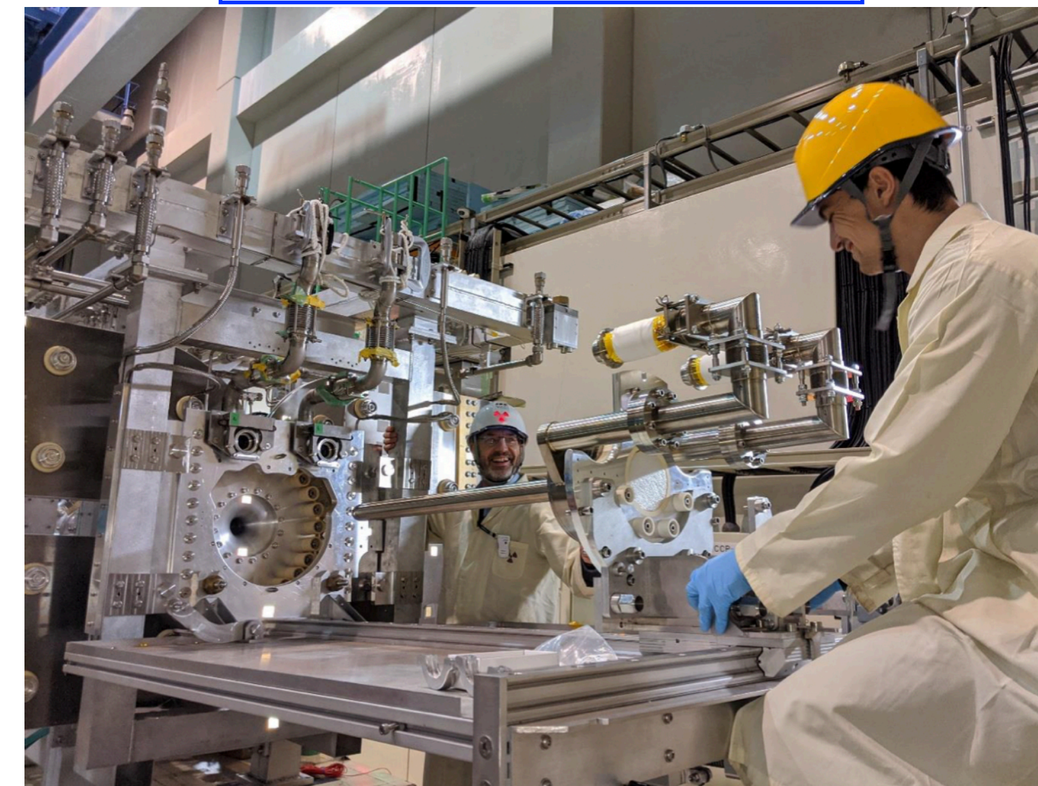
Target installation to new Horn1
