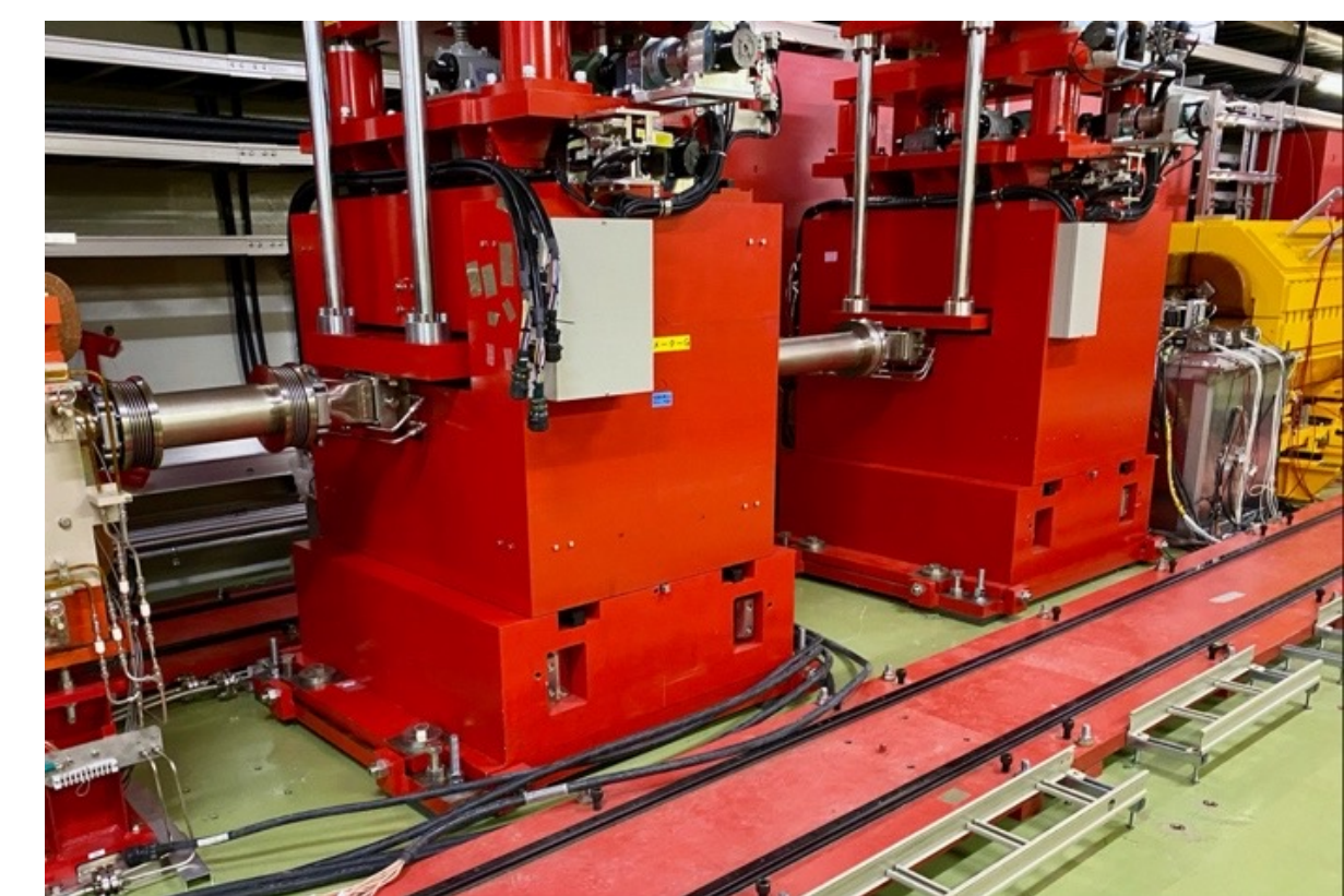
Newly installed Col. G Col. H
