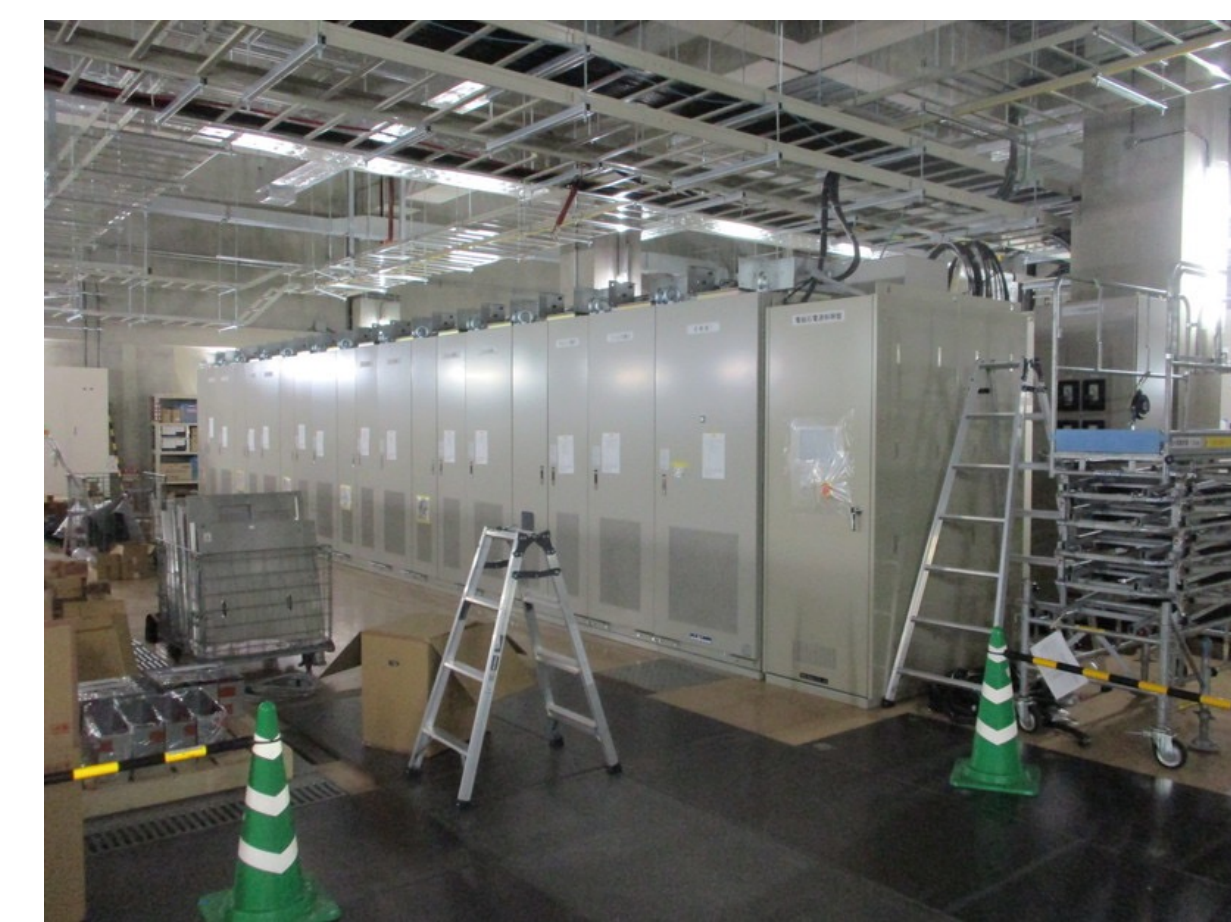
QDN power supply (Chopper + Filter + Control Panels)
