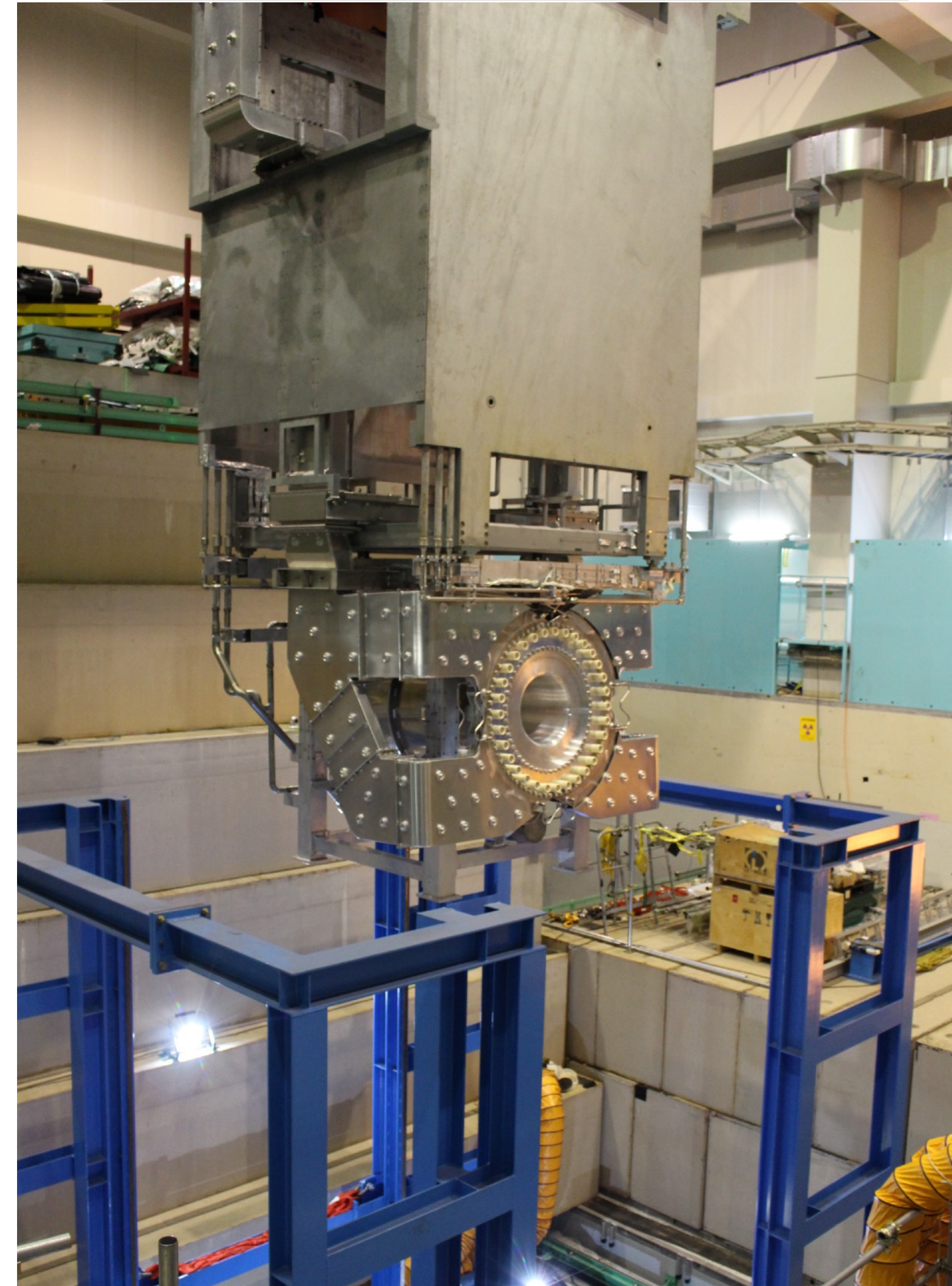
New Horn2 (3rd gen.) installation
