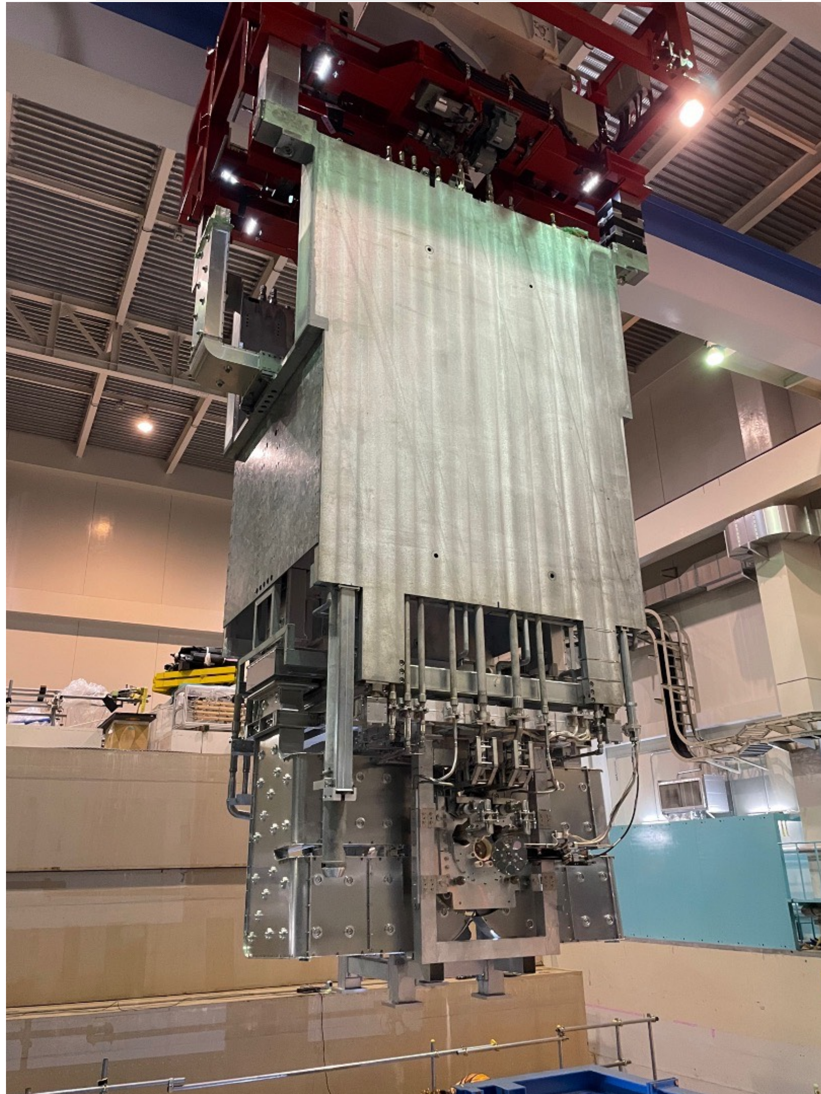
New Horn1 (3rd gen.) installation
