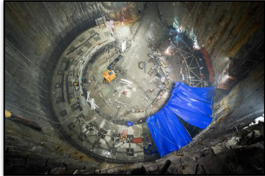
Excavation of the pool
