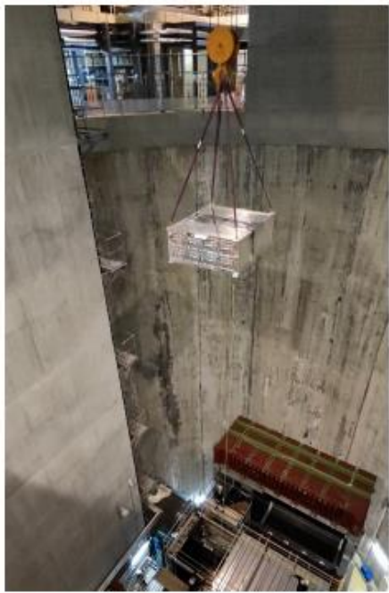
Bottom TPC installation (September 2023)
