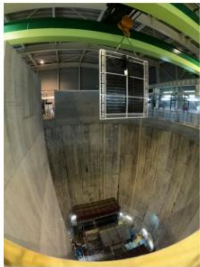
TOF installation (July 2023)
