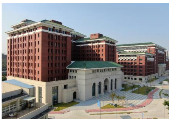
Haiqin 5 th building
