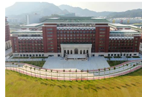
Haiqin 4 th building
