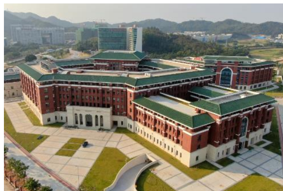
Haiqin 6 th building
