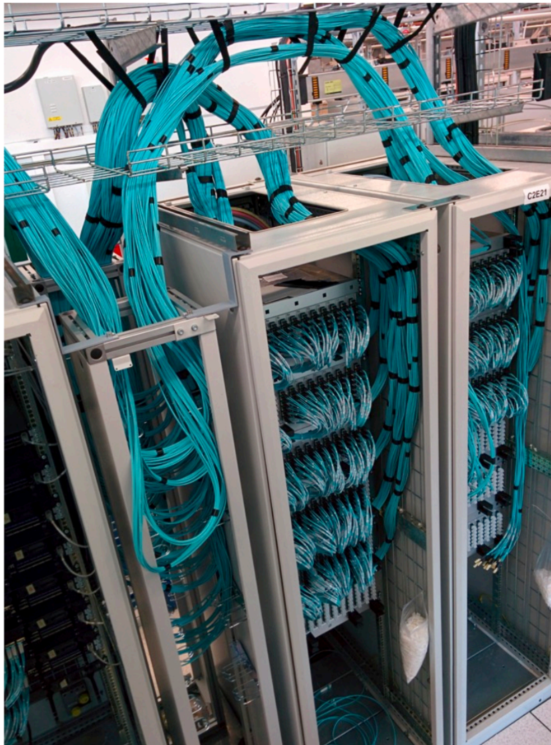
CMS Data concentrator 'patch panels' and switches
