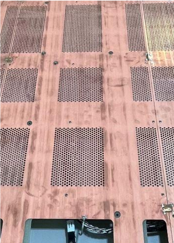
new version covering the cables in the composite openings
