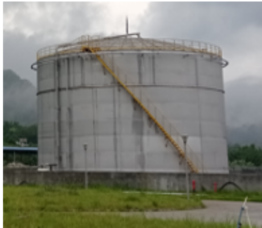
5000 m 3 LAB storage tank
