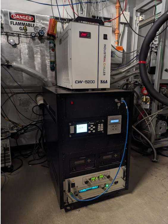
D-D generator control rack.
